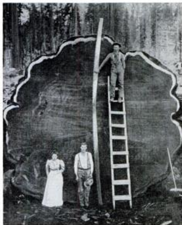
Crosscut saw for the big trees was a long ribbon of steel made by welding two ordinary saws end to end
